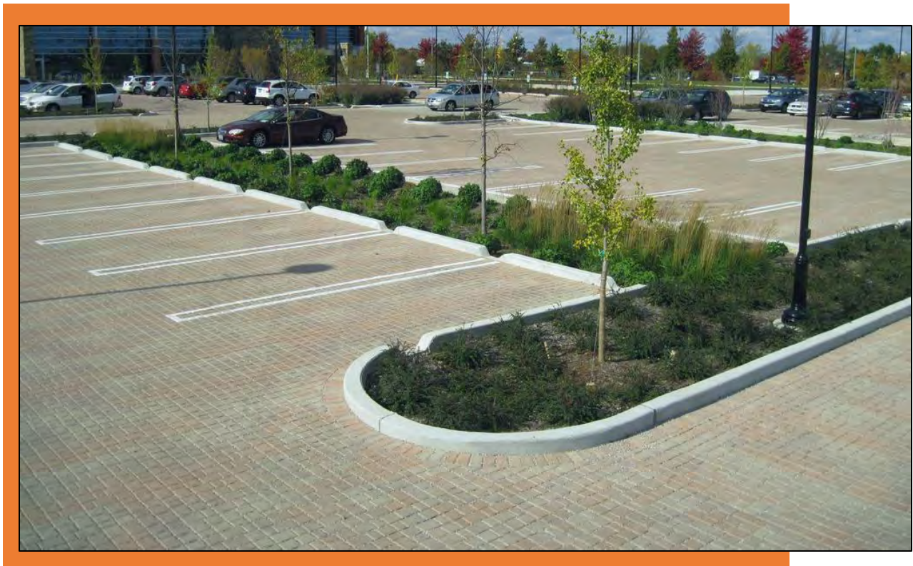
Figure 3.406-1: A permeable surface used in combination with a rain-garden.
