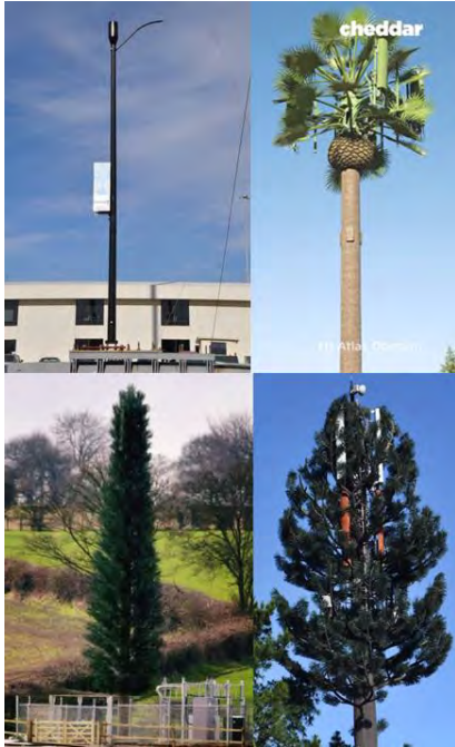
Figure 3.205-2 Stealth Technology for Small Cell Towers
